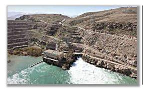
The Kajaki Dam is in the north of Helmand Province. It was commenced in the 1950s, with the hydroelectric plant started in the 1970s by US Aid. In partial completion, it was abandoned in 1979 during the Russian invasion. Only two if its three turbine units have ever been operational, with frequently only one working. In 2008 a third 220-tonne turbine was delivered during a high-intensity operation, which was hailed by NATO as a significant victory. The turbine remains non-operational.
